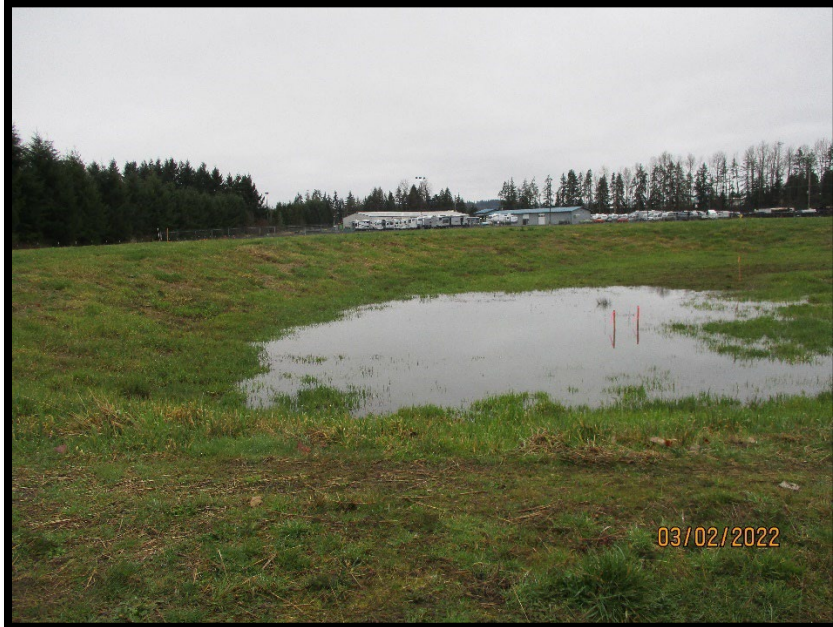
Photograph 6: Constructed storm water collection pond in the southwest corner of the subject site. Photo is looking north near the western property boundary.
